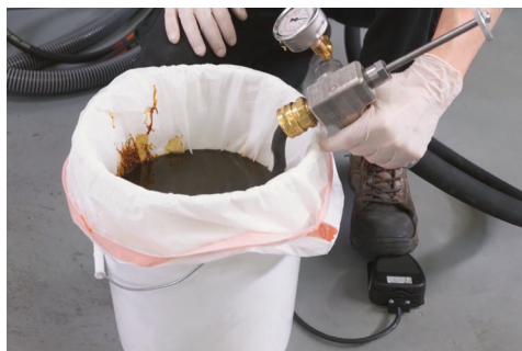
23) Hold the fill hose over a suitable container and run the mixture through the entire fill hose and gun to ensure proper flow. Here we used the foot switch to run the machine.
