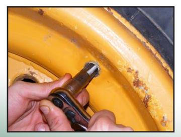
After the valve stem port has been enlarged, run the 3/8 inch tap into the hole to cut the threads.
