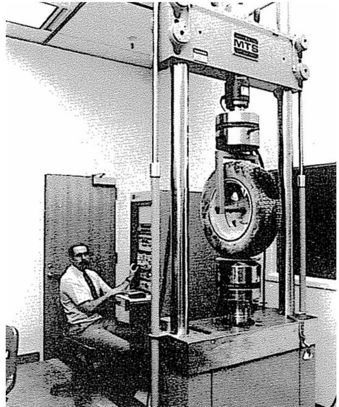
Fig. 21- Unwrapped tire on MTS test equipment; oval dark spot in frost on tread was produced by previous test, tire rotated 120°
