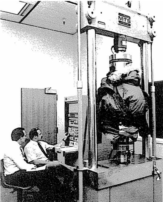
Fig. 20 – Thermally insulated tire in MTS equipment on which load deflection curves were run after chilling to -40°F
